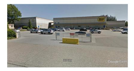
This was a "Tilt-up" concrete design for five (5) acres in size. It was certainly the type of contract that my partners, Rempel wanted me to pursue for it was essentially a concrete building with steel post, beam, truss, and steel deck roof construction.
