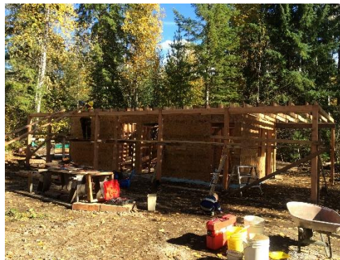
Ceiling Joists Under Construction
