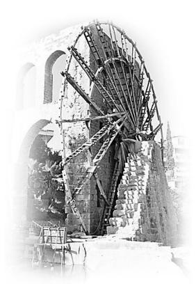
water pump. The river that provides the water it raises also serves as its sole source of energy.
