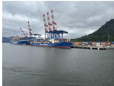
PR modern Dock Loading facilities for railcar and ship
